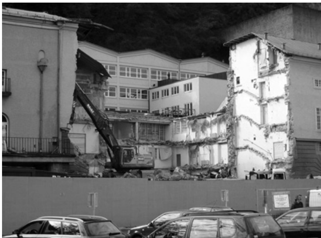
Salzburg, Neues Festspielhaus, demolition in October 2004
